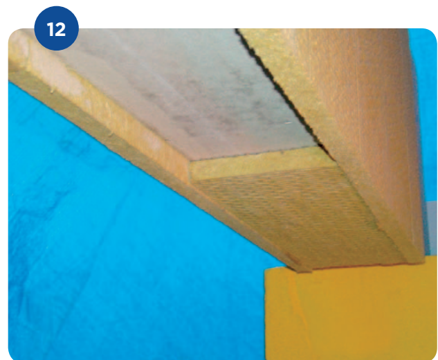
The flange is glued in the end
