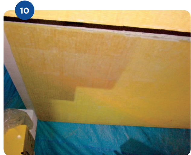
Finished ORDEXAL® B lining
