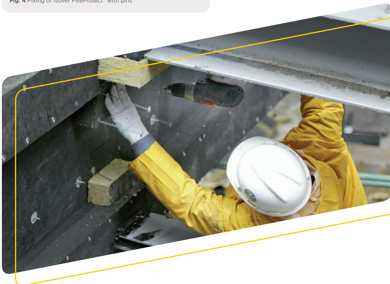
Fig. 4 Fixing of Isover FireProtect® with pins
