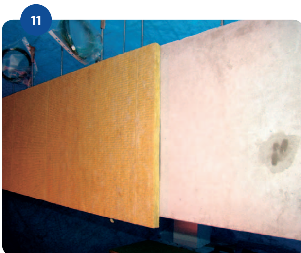
In case of a beam, the sides are glued first
